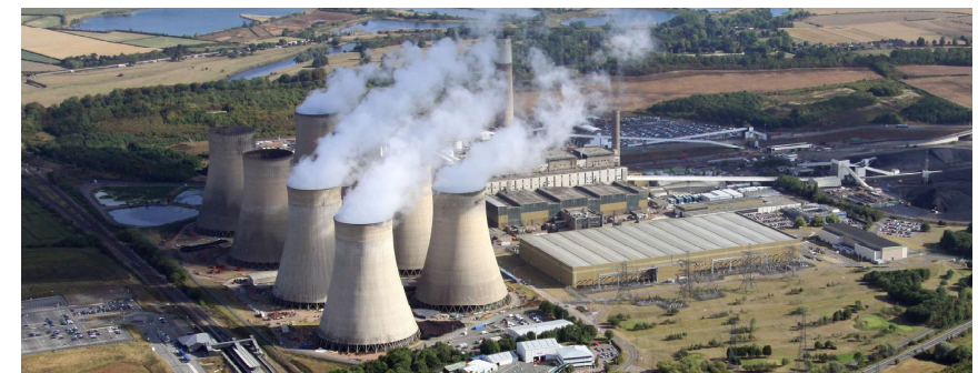
Aerial view of the site's Northern Area
