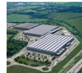
Example of car batteries factory
